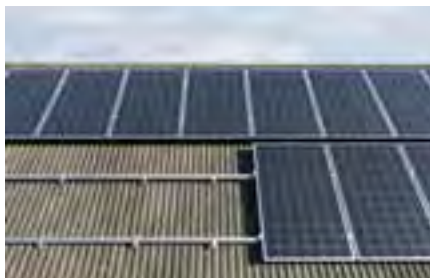
Pitched roof with corrugated sheets covering
