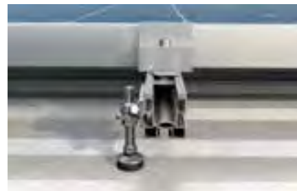
Roof with trapezoidal metal sheet covering
