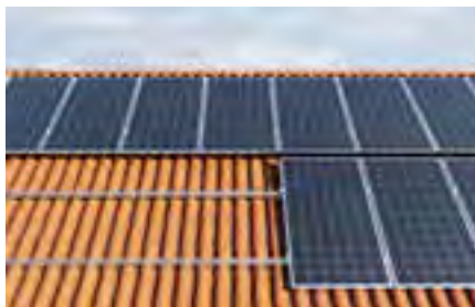
Pitched roof with tiles
