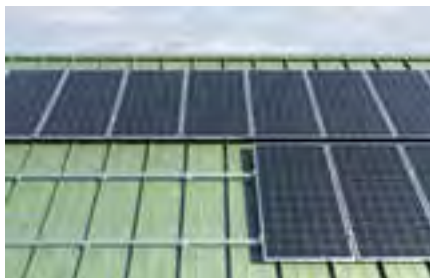
Pitched roof with flat standing seam covering
