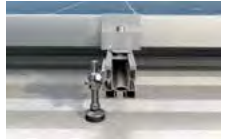
Roof with trapezoidal metal sheet covering
