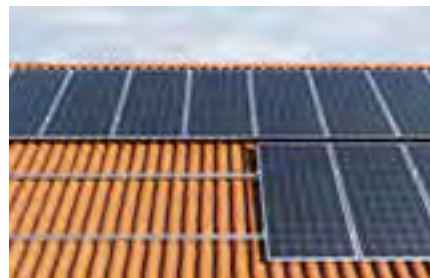
Pitched roof with tiles
