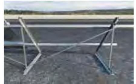
Mounting detail on a flat roof
