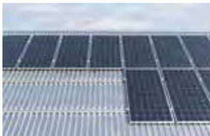
Roof with trapezoidal metal sheets covering
