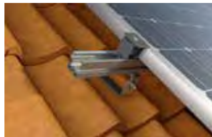
Pitched roof with tiles
