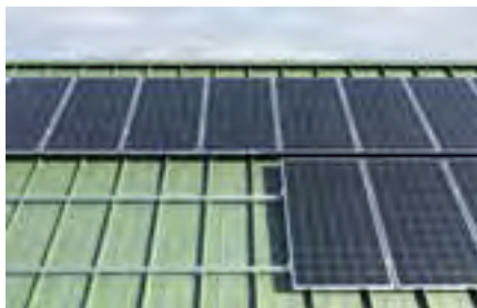
Pitched roof with rounded standing seam covering
