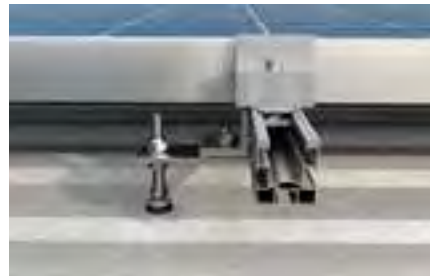
Roof with trapezoidal metal sheet covering
