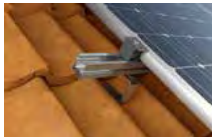
Pitched roof with tiles
