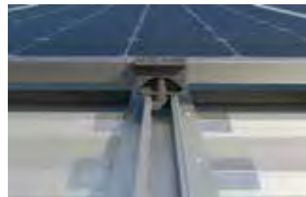
Roof with trapezoidal metal sheets covering
