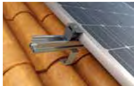
Pitched roof with barrel tiles
