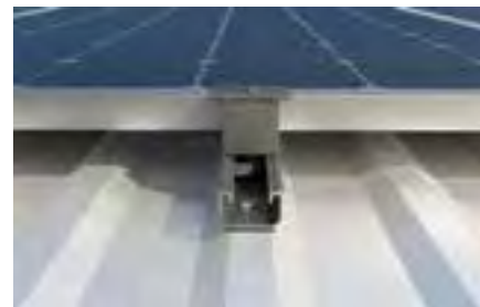
Roof with trapezoidal metal sheets covering
