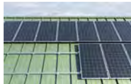
Pitched roof with flat standing seam covering
