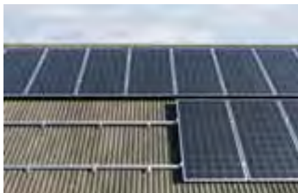
Pitched roof with corrugated sheets covering
