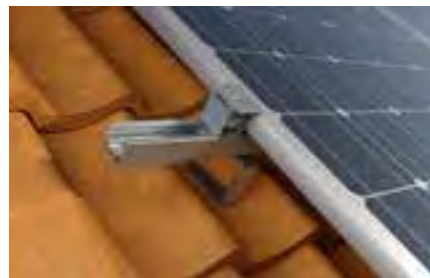
Pitched roof with tiles
