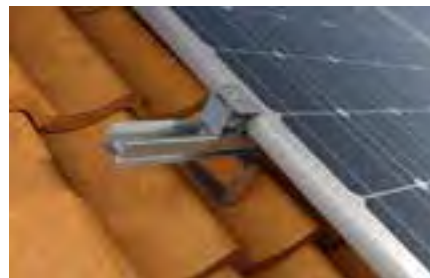
Pitched roof with tiles
