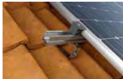
Pitched roof with tiles - RH HB A2
