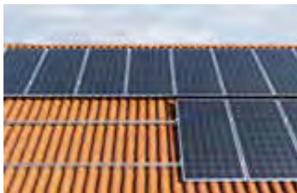
Pitched roof with tiles
