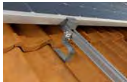
Pitched roof with tiles
