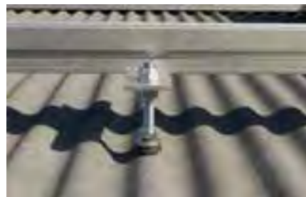
Pitched roof with corrugated sheets covering
