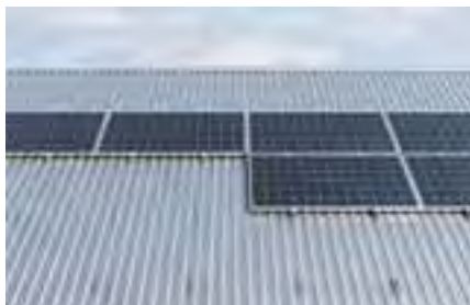
Roof with trapezoidal metal sheets covering
