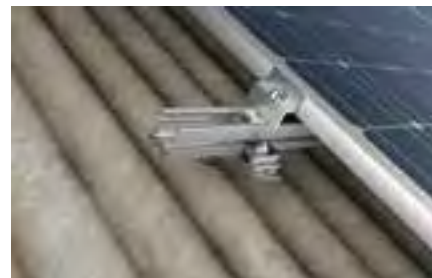
Installation rail with SSP Speed Plus A2
